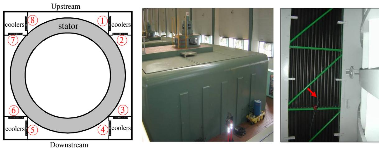
Figure 5: Ozone monitoring location inside Shipshaw generators enclosure.
